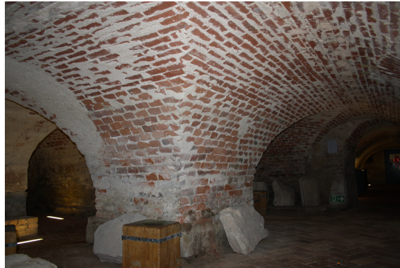
Fig. 6 Basilica Nanebevzetí Panny Marie in Velehrad (Czech Republic) - underground built of baked bricks in the 17th century on the foundations of the 13th century (photo P. Hronček)
