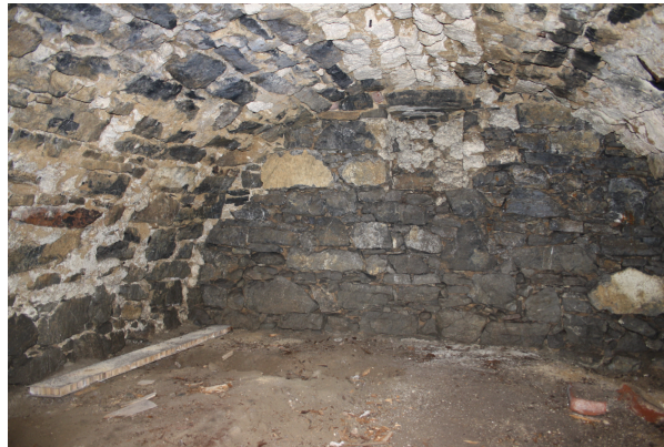
Fig. 5 Cellar in Brusno (18th century), built partially worked quarry stone connected with lime mortar (photo P. Hronček)
