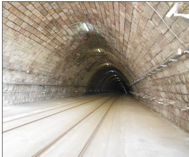
Fig. 7 Bratislava (tramway) tunnel built of worked stone blocks (1949) (photo P. Hronček)
