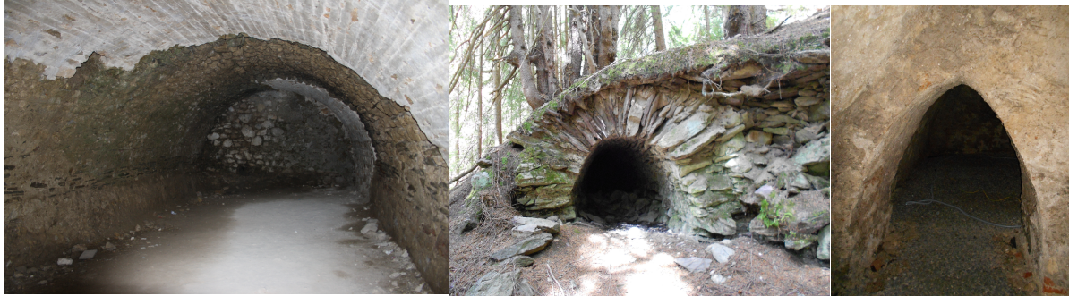
Fig. 2 The cylindrical barrel vault, cellars of the castle Čachtice (15th century) (left), Elliptical barrel vault, the water adit (tunnel) in Špania Dolina (16th-17th century) (middle), Broken (Gothic) barrel vault underground of the castle Slovenská Ľupča (18th century) (right side of the Fig. 1) (Photo P. Hronček)
